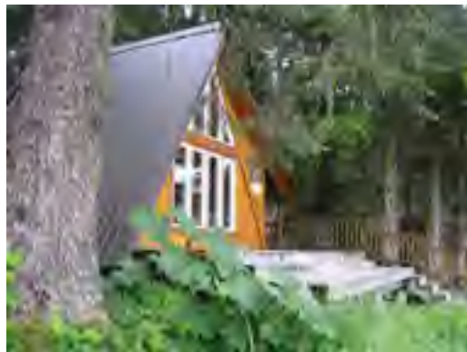
Photo 4-2. West Point Cabin
